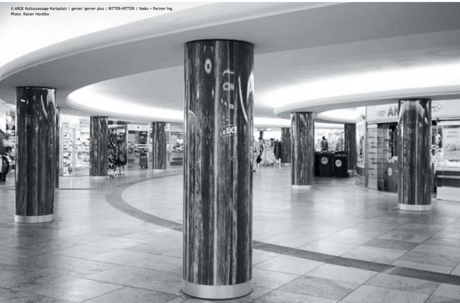
Column design for Kulturpassage at Karlsplatz, Vienna, Austria: Bent white glass laminated with printed PVB and backed with TROSIFOL® Diamond White
