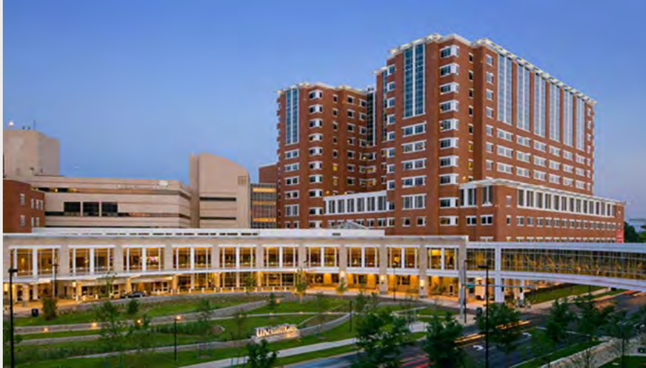
University of Kentucky Hospital Unitized curtain wall and punched openings with Super Spacer Triseal
