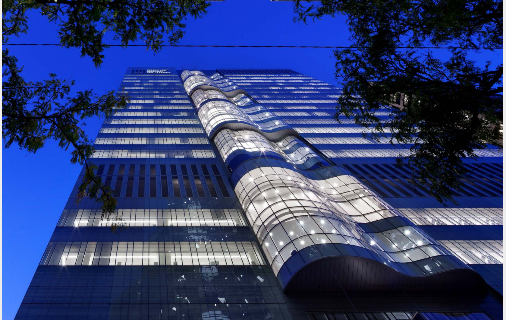
Sick Kids Hospital, Toronto ON 20 Stories of Bent IG with Super Spacer Triseal Architect: Diamond Schmitt
