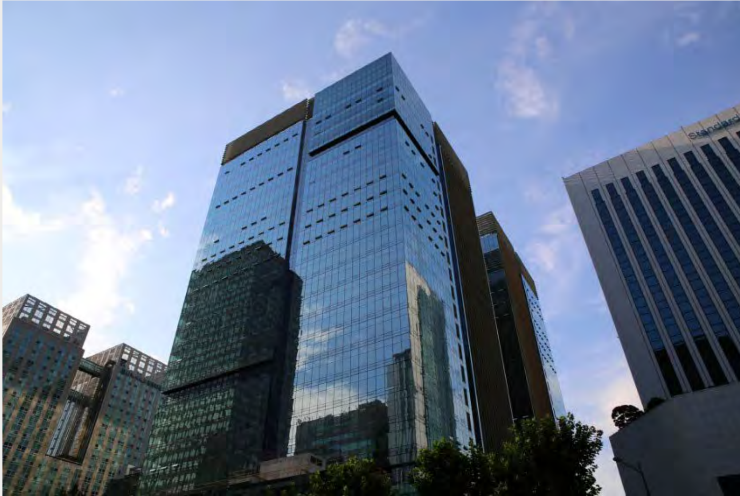
GS Jongro Tower , Seoul, South Korea ~400,000 Square feet of SSG Super Spacer Triseal IG Architect: Changjo
