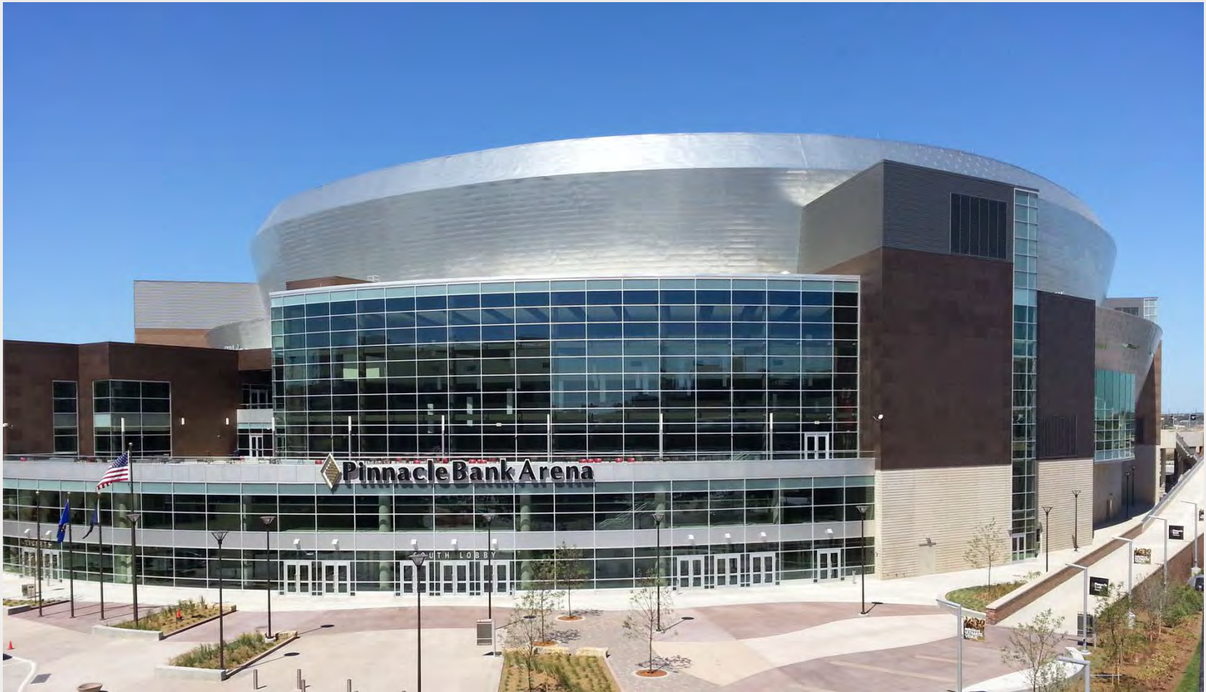
The Pinnacle Bank Arena, Lincoln, NE 40, 000+ Sq ft of Super Spacer Triseal Architect: DLR and BVH
