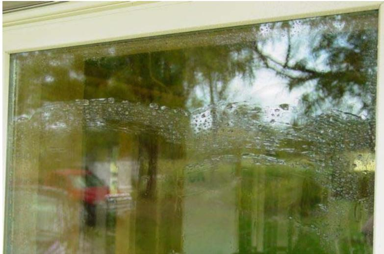
2. To remove contaminants from the glass surface take a small amount of Cerium Oxide powder and place in a small cup. Mix with tap water to form a paste with the consistency slightly less than motor oil. Thin the mixture as needed by adding more water.
